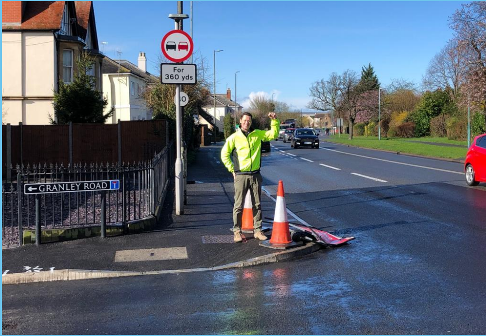
[Stretch of A40 by Granley Road that has just been resurfaced.]
